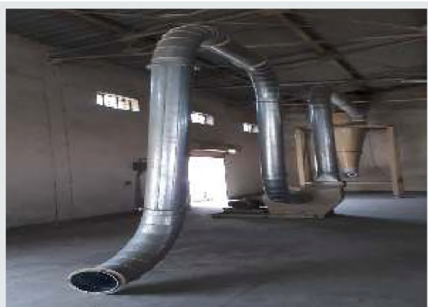
Trash handling system to control pink bollworm in cotton ginneries
