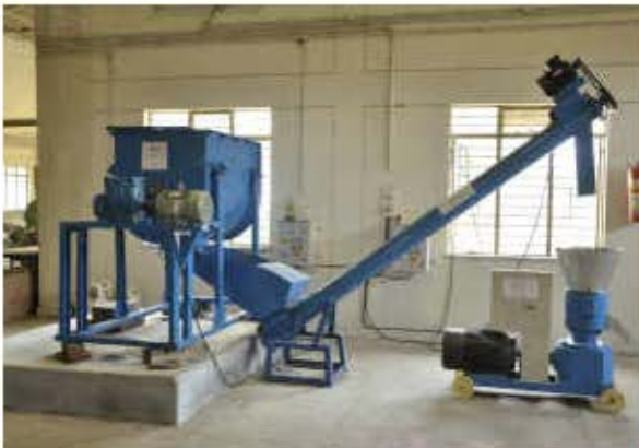
Cotton stalk pelleting unit installed at GTC, Nagpur
