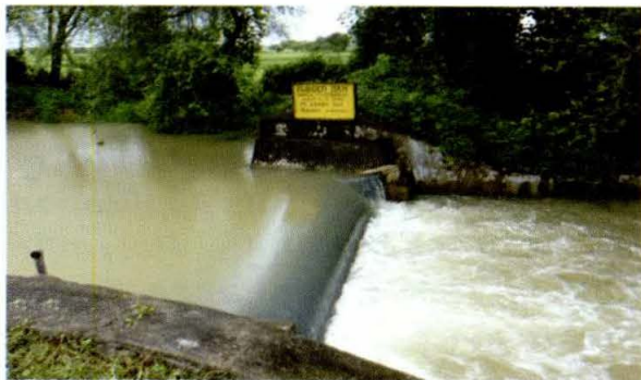
Fig. 7. Rubber dam at Baghamari D/W - 4 Watershed, Odisha
