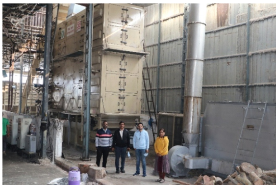
Fig. 1.2.1 Continuous feeding cottonseed dryer at Shree Krishna Cotton Company, Saoner, Nagpur
